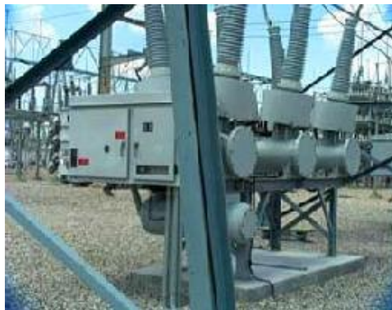
Gambar 2.4 SF6 Circuit Breaker
