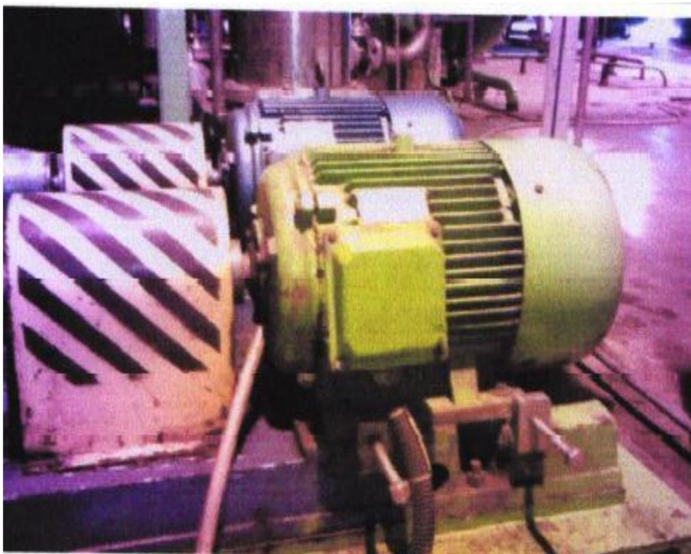
Gambar 2.2 Mesin *Generator Stator Cooling Water Pump #20B*
