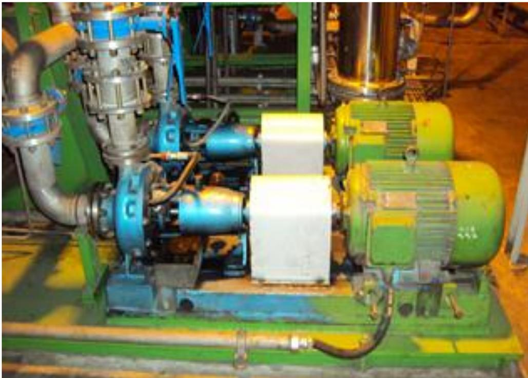
Gambar 2.3 Motor *Generator Stator Cooling Water Pump A*
