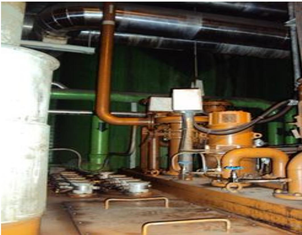
Gambar 2.4 *Motor Lube Oil Bfpt Pump*
