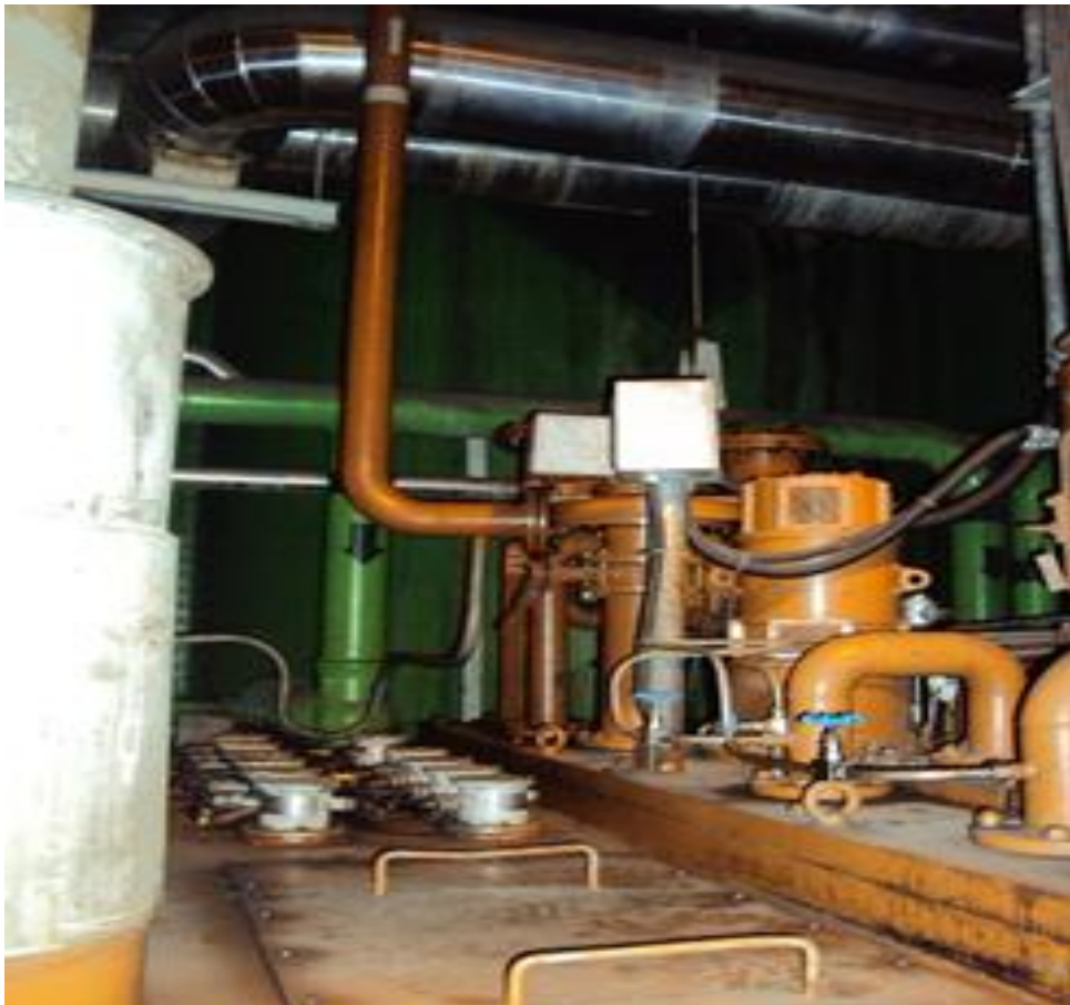
Gambar 4.1 Motor Lube Oil Bfpt Pump
