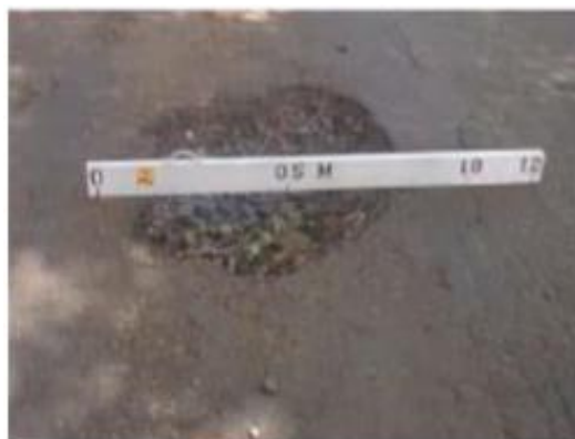
Gambar 3.26 Lubang ( Pathole )
