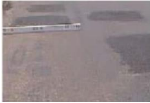
Gambar 3.22 Tambalan ( Patching end Untiliti Cut Patching )
