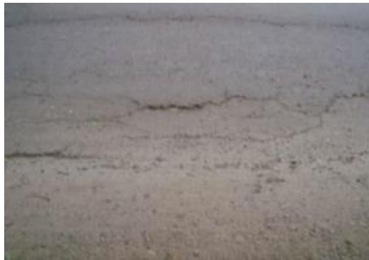
Gambar 3.8 Cekungan ( Bumb and Sags )
