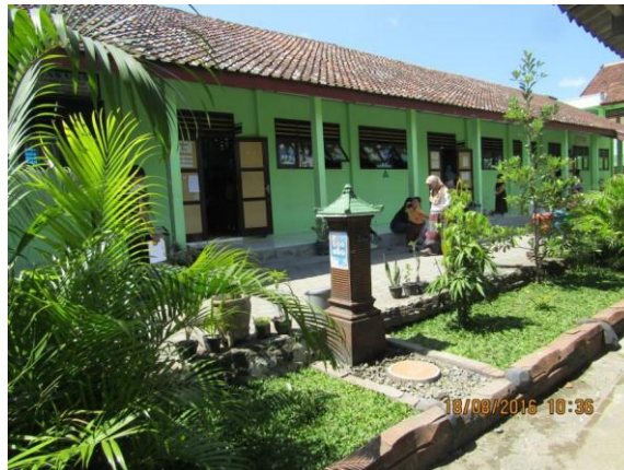
Gambar 2.1 Tampak depan SD kaligondang Faizah, et.al. (2017)
