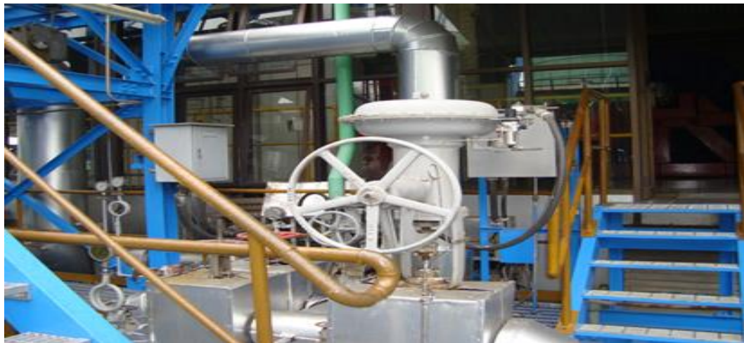
Gambar 2.9 Ejector First Stage
