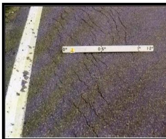
Gambar 3.18 Slippage cracking .
