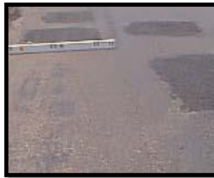
Gambar 3.12 Patching and utility cut patching.
