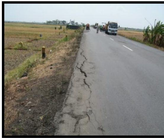
Gambar 3.8 Edge cracking .
