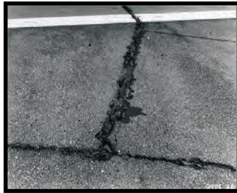
Gambar 3.9 Joint reflection cracking .
