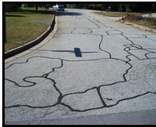
Gambar 3.4 Block cracking .
