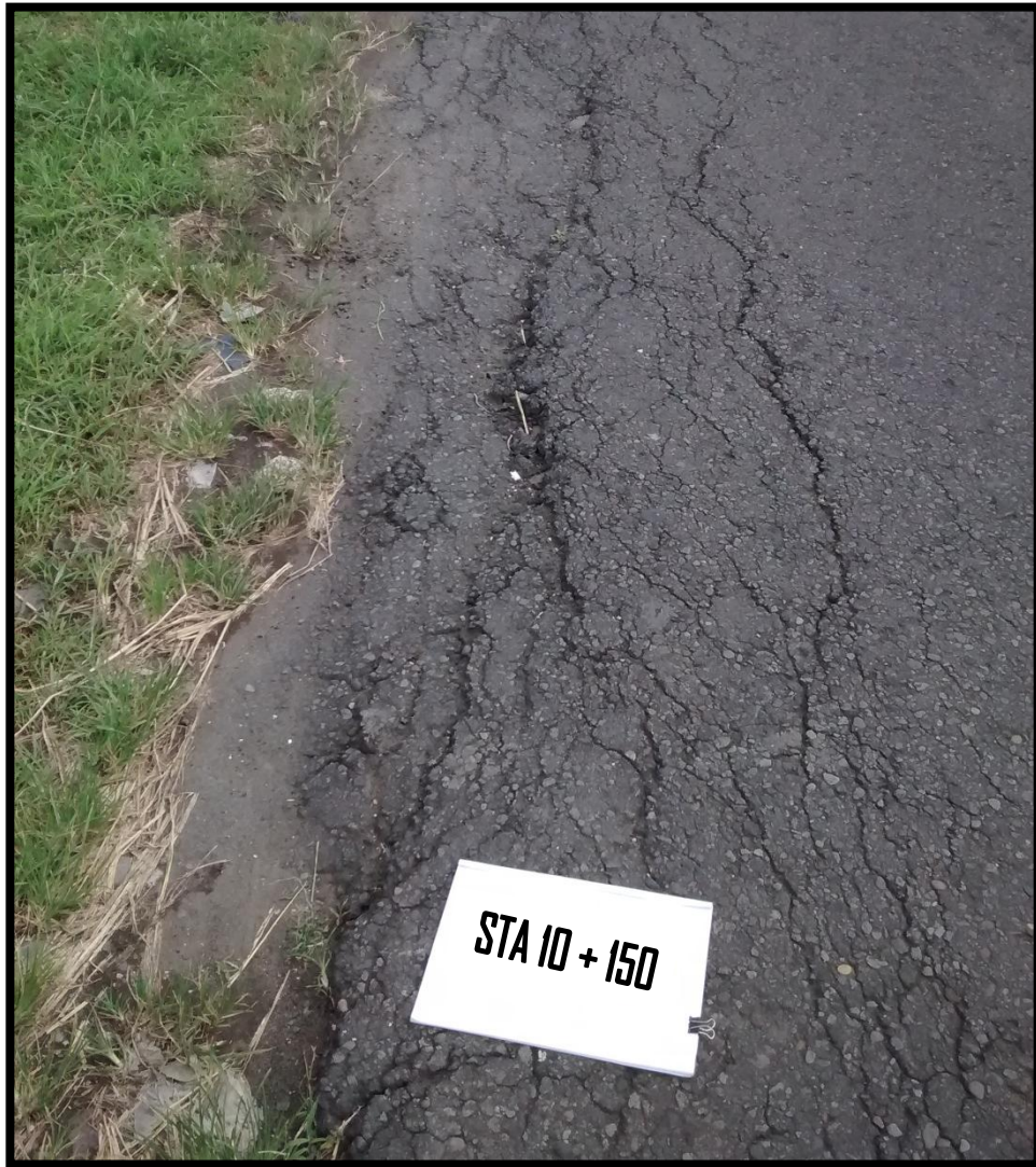
Gambar 11. Patah slip.
