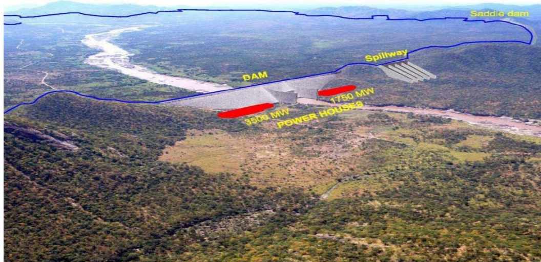
Figure 4: Aerial Photograph of the GERD Construction area
