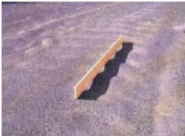
Gambar 2.13 Keriting ( Corrugation ) Sumber : Bina marga no.03/MN/B/1983
