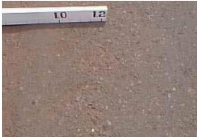
Gambar 2.27 Pengausan Agregat ( Polised Agregat ) Sumber : Bina marga no.03/MN/B/1983
