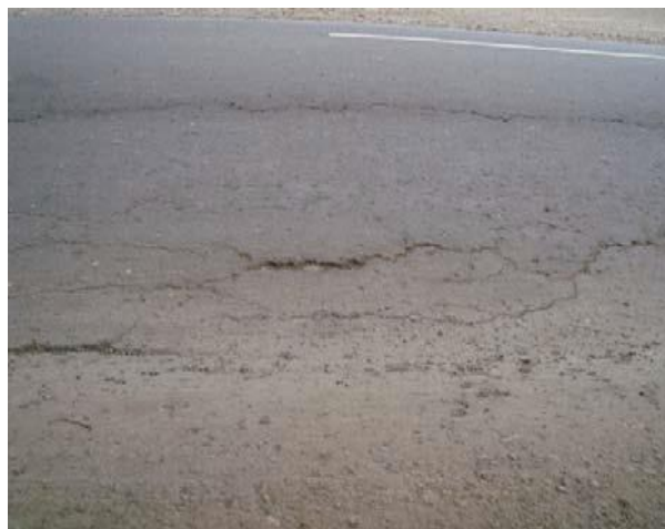
Gambar 2.11 Cekungan ( Bumb and Sags )
