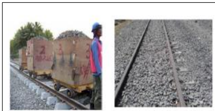
Gambar Error! No text of specified style in document..36 Penghamparan upper-ballast
