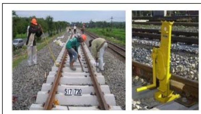
Gambar Error! No text of specified style in document..34 Pemasangan penambat rel
