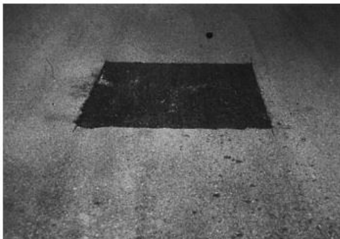
Gambar 3.21 Tambalan ( Patching and Utility Cut Patching )
