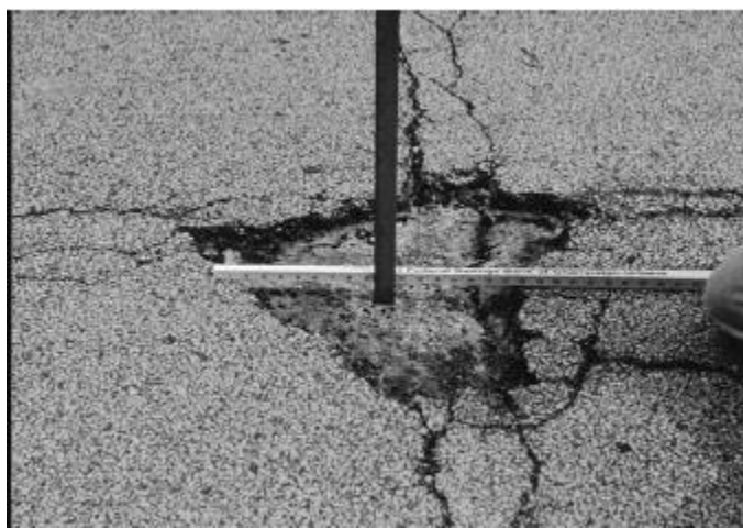
Gambar 3.25 Lubang ( Pothole )
