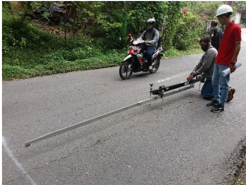
c. Proses Pengaturan Alat Benkelman Beam
