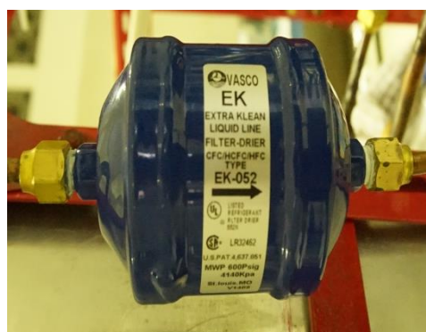
Gambar 3.22 Filter Dryer
