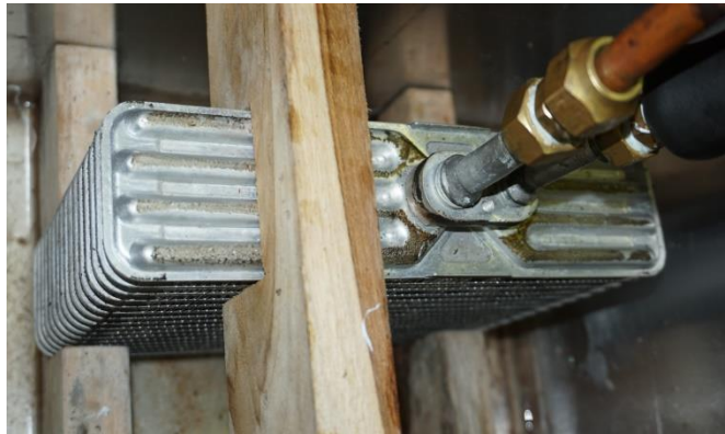
Gambar 3.8 Evaporator
