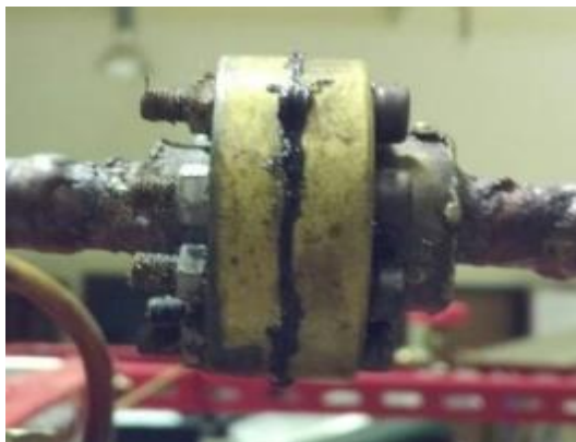
Gambar 3.24 Orifice
