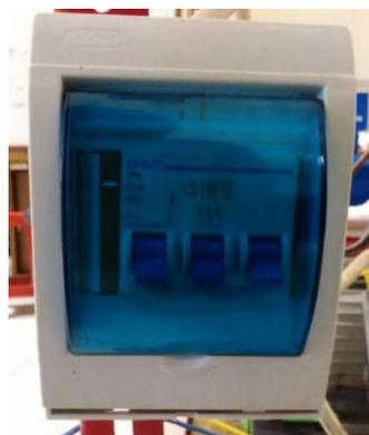
Gambar 3.13 *MCB (Mini Circuit Breaker)*
