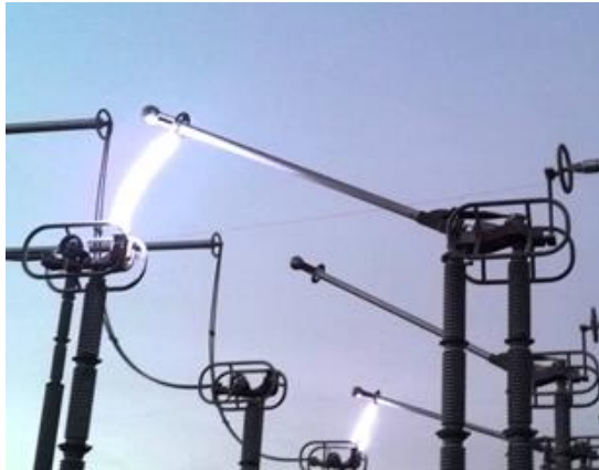
Gambar 2.4 Disconnecting Switch
