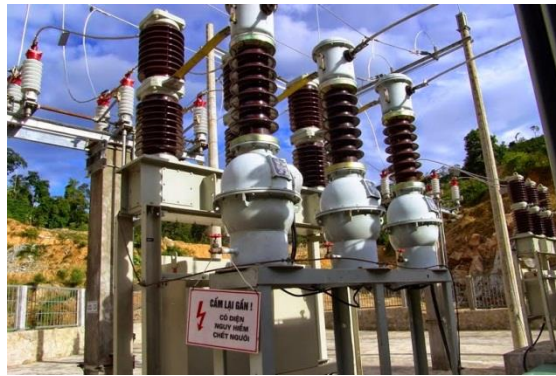
Gambar 2.6 Current Transformer
