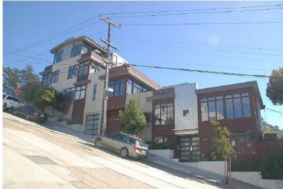
Gambar 2.4 Contoh Sloping Site ( Sumber : FEMA P-154 2015 )
