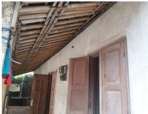
Gambar 4.24 Rangka atap material bambu ( Sumber : Survei Lapangan 2018 )
