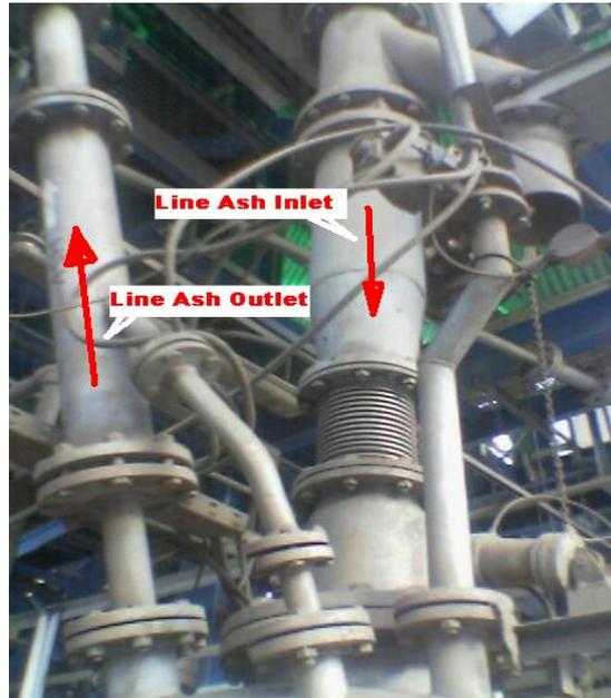
Gambar 2.18 Line Ash Inlet dan Line Ash Outlet
