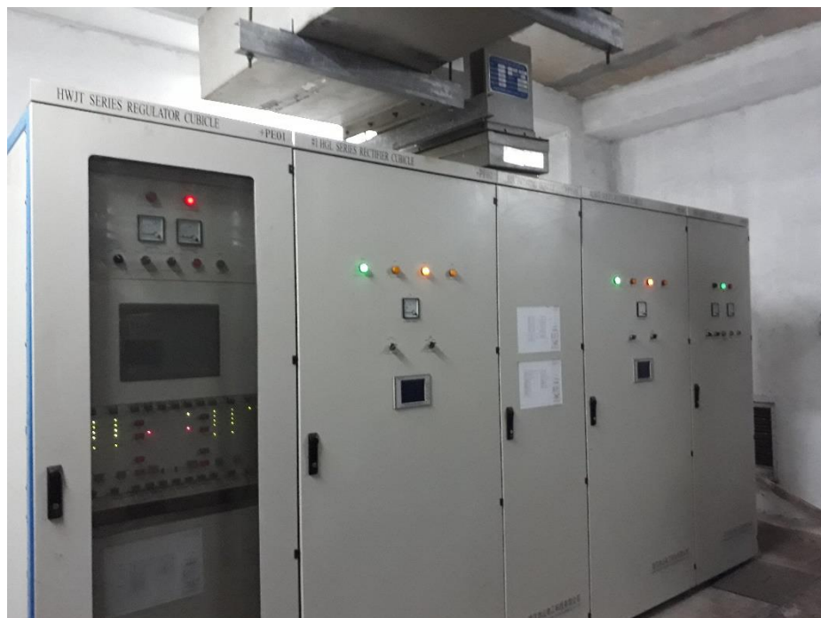
Gambar 4.3 Motor Control Center
