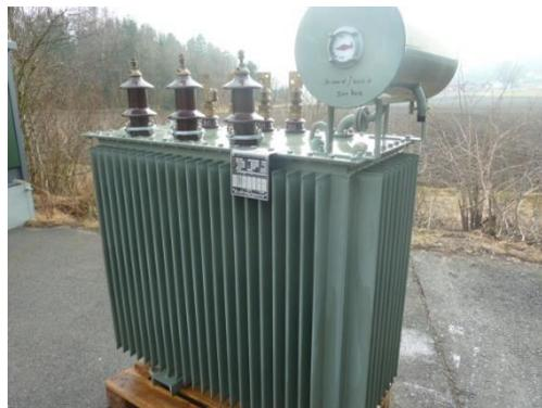
Gambar 1.5 Transformator distribusi step down 500 kVA
