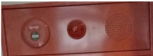
Gambar 13 Alarm manual
