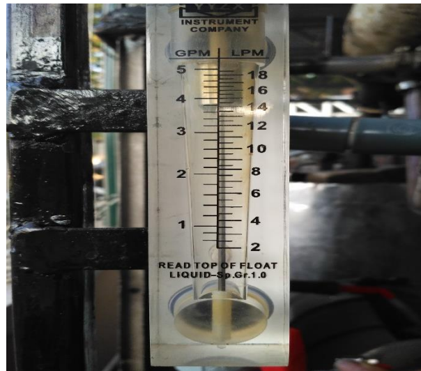
Lampiran 3 Flowmeter debit 18 LPM
