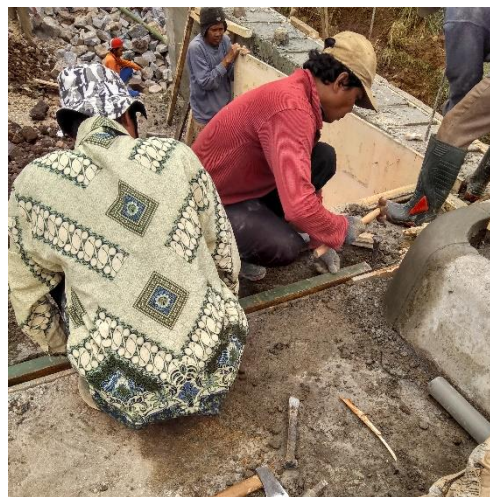
Gambar 4.20 Pemasangan expansion joint
