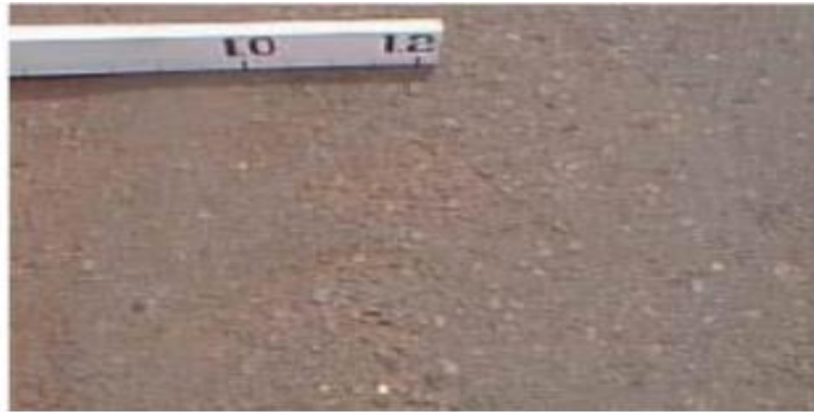
Gambar 2.27 Pengausan Agregat ( Polised Agregat )
