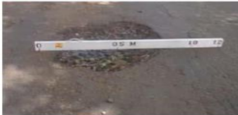
Gambar 2.29 Lubang ( Pathole )
