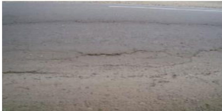
Gambar 2.11 Cekungan ( Bumb and Sags )
