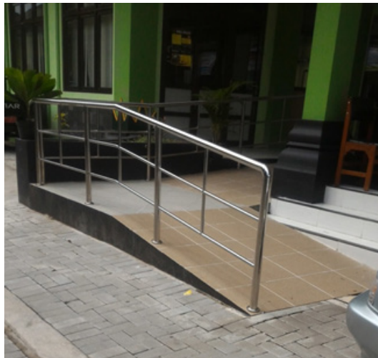
Picture 6. Ramp in Wirobrajan sub-District Office
