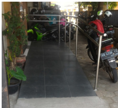
Picture 2. Ramp in People Central Health Wirobrajan Sub-district
