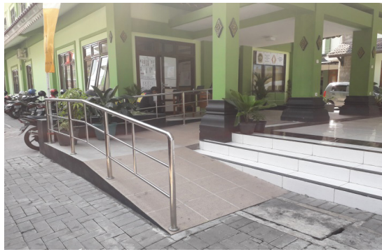
Picture 1. Ramp in south side Wirobrajan Sub-district Office
