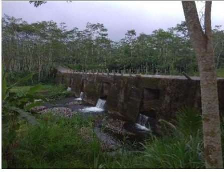
Gambar 9 Sabo Dam S6
