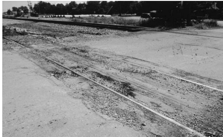
Gambar 2. 33 Rusak perpotongan rel (ASTM, 2007)
