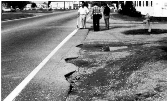
Gambar 2. 19 Retak pinggir ( edge cracking ) (ASTM, 2007)
