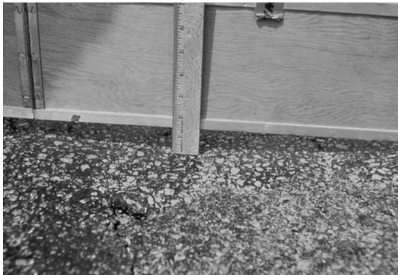
Gambar 2. 35 Kerusakan alur ( rutting ) (ASTM, 2007)
