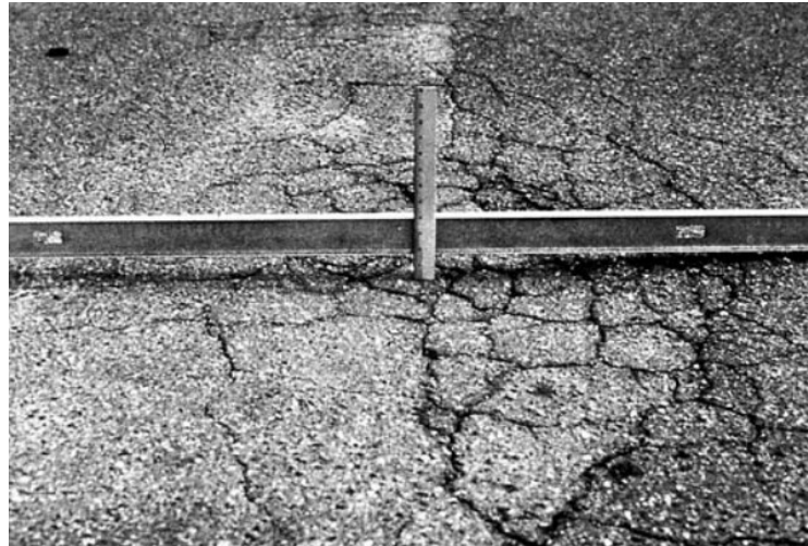
Gambar 2. 17 Amblasan ( Depression ) (ASTM, 2007)
