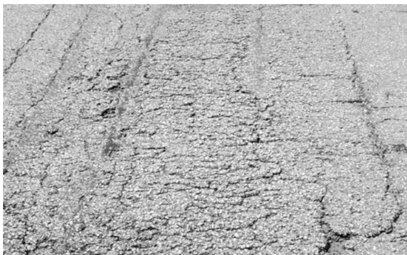
Gambar 2. 43 Pelepasan butir (ASTM, 2007)
