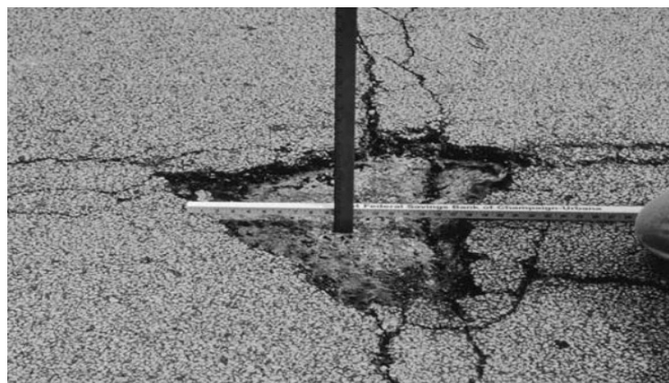
Gambar 2. 31 Lubang ( Pothole ) (ASTM, 2007)
