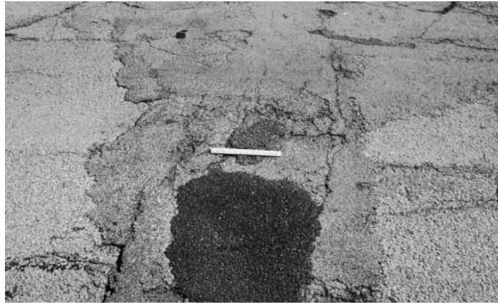
Gambar 2. 27 kerusakan tambalan (ASTM, 2007)
