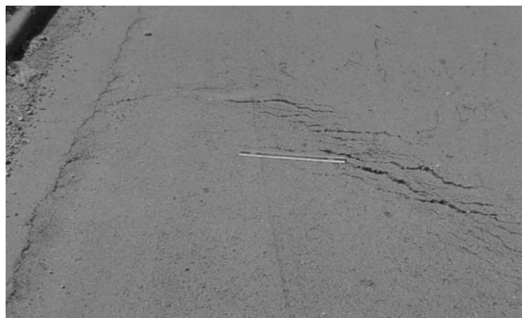
Gambar 2. 39 Patah slip (ASTM, 2007)
