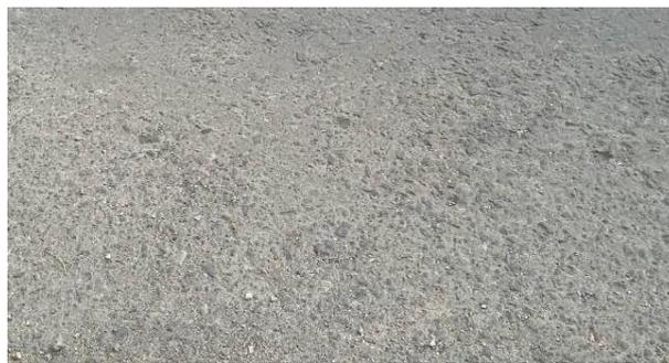
Gambar 2. 27 Pengausan Agregat (*Polished Aggregate*)
