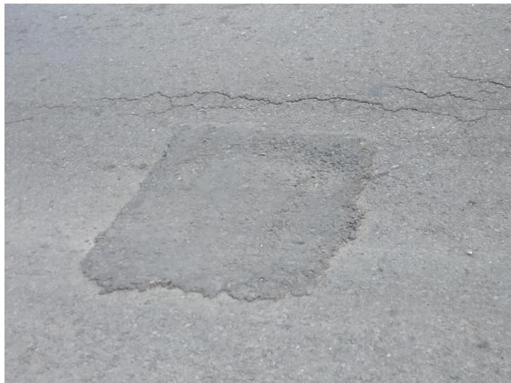
Gambar 2. 33 Tambalan (*Patching and Utility Cut Patching*)
