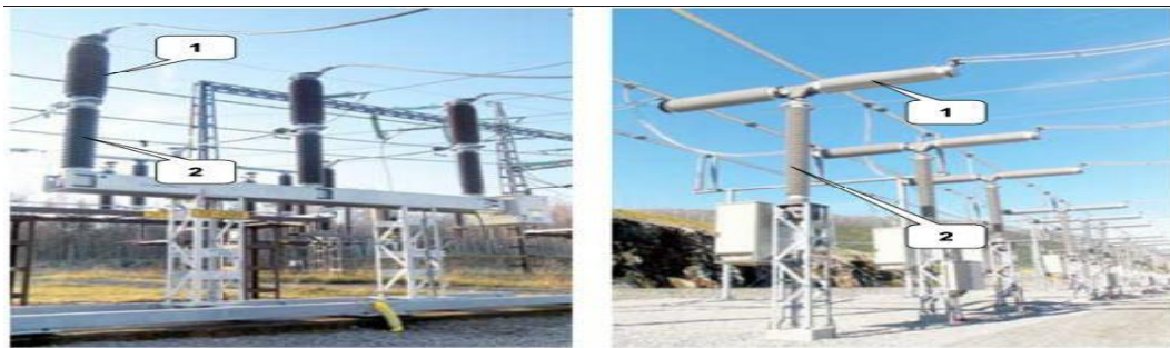
Gambar 2.6 Isolator interrupting Chamber dan Support
