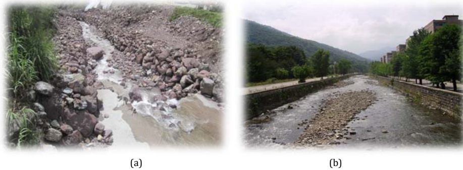
Figure 13. (a) Normalization using natural rocks, (b) Normalization using vertical gabions
