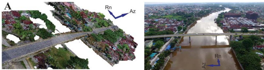
Figure 3. Location of Siak Bridges taken by Small UAV for Siak Bridge I.
