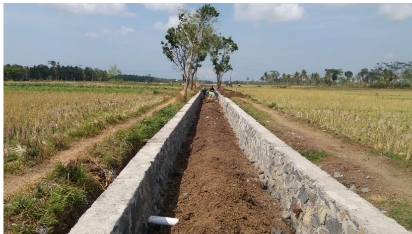
Picture 3.1 Program of Irrigation and Sewers Construction
