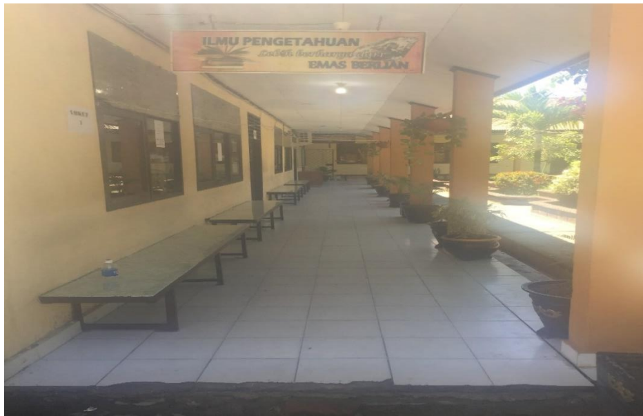
Figure 3.5 condition of hallway to the class at SMAN 4 Kota Palu
