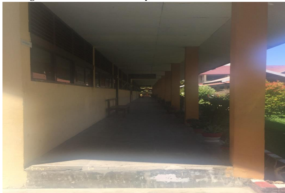
Figure 3.6 condition of hallway to the class at SMAN 4 Kota Palu
