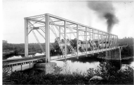
Gambar 1 Contoh jembatan rangka (Unsworth, 2017)
