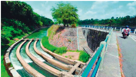
FIGURE 8: Another side view of irrigation canal in Bligo village, Ngluwar district, Magelang regency, Central Java province, Indonesia.
