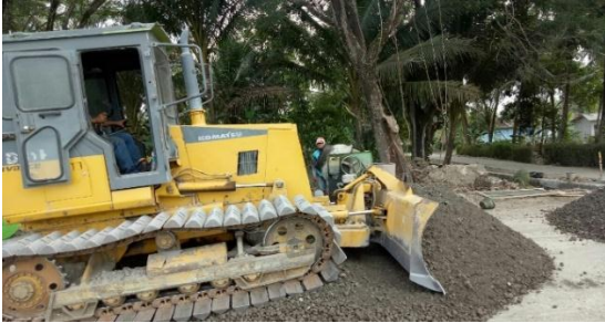
Gambar 3 Pekerjaan CTB ( Cemen Treatment Base )
