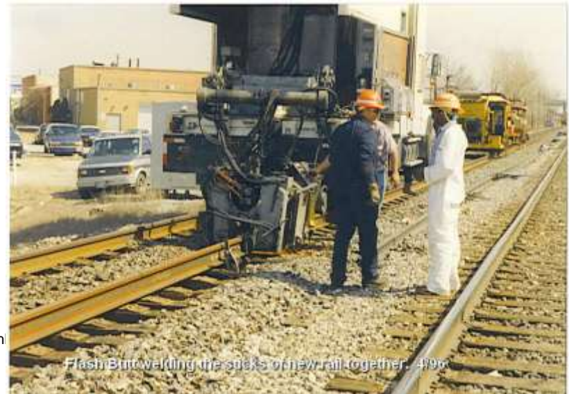
http://www.railroad.net/santucci/Flash_Butt_Welding.jpg
