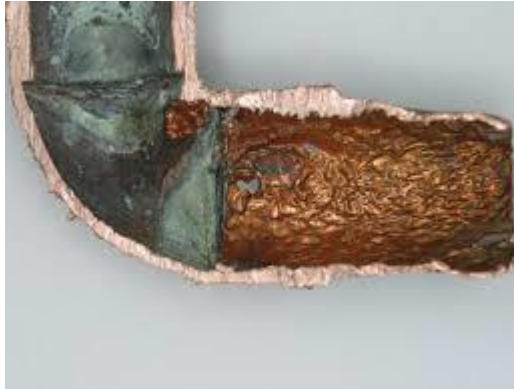
Gambar 2.8 Korosi Erosi (Mechanicalengineering, 2014)
