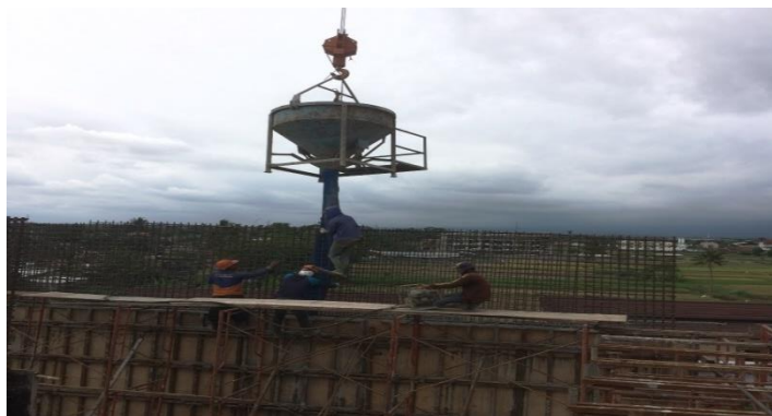
Gambar 4.9 pengecoran shearwall
