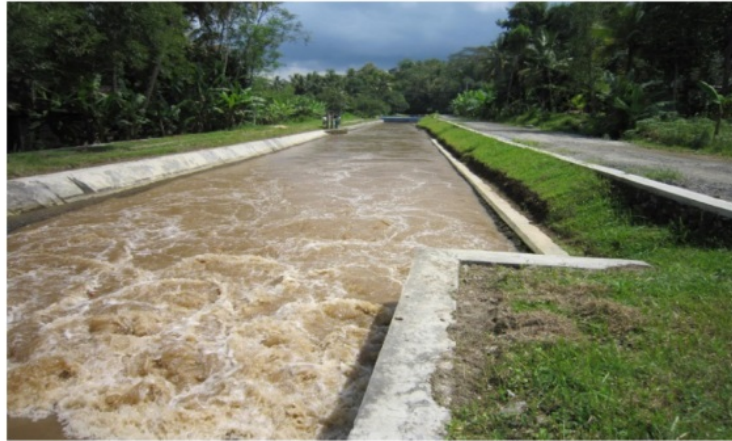
Fig. 1. Irrigation canal in Semawung, Banjarharjo Village, District of Kalibawang, Kulon Progo Regency, Special Region of Yogyakarta.
