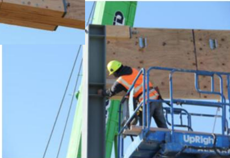
Figure 10: Installer completing the Quick Connect joint by placing bearing plate and tightening nut on main tension rods
