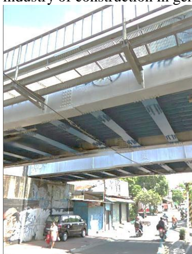
Figure 1. Examples of steel usage as inspection way at briges in Yogyakarta
