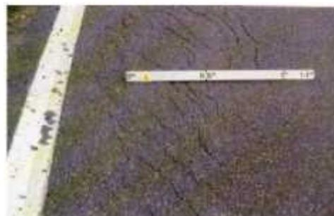
**Gambar 3.35** Patah Slip (*Slippage Cracking*)
