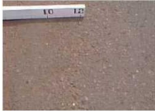
**Gambar 3.25** Pengausan Agregat (*Polised Agregat*)
