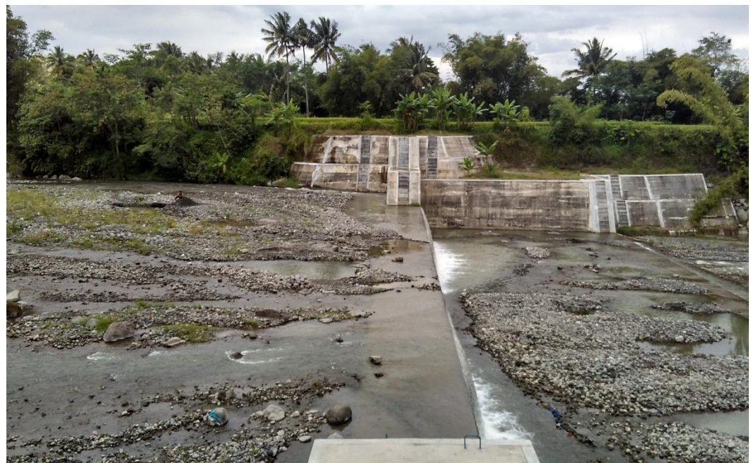
Tampak Samping Sabo Dam
