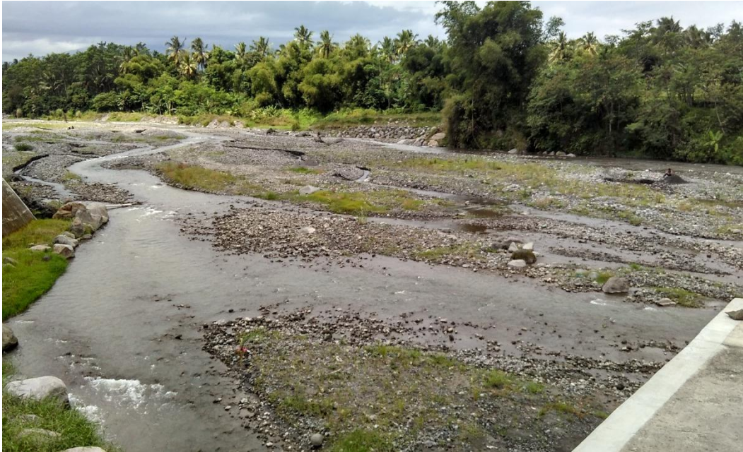
Tampak Bagian Hulu Sabo Dam
