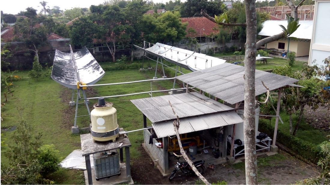
*Gambar Sistem Solar Parabolic Through Collector*
