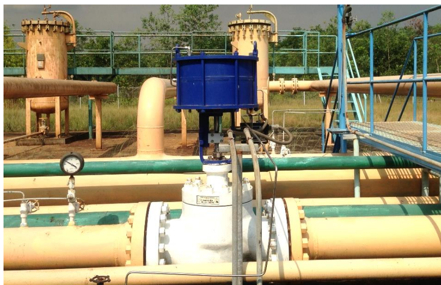
Gambar 3.9. Control valve north header
