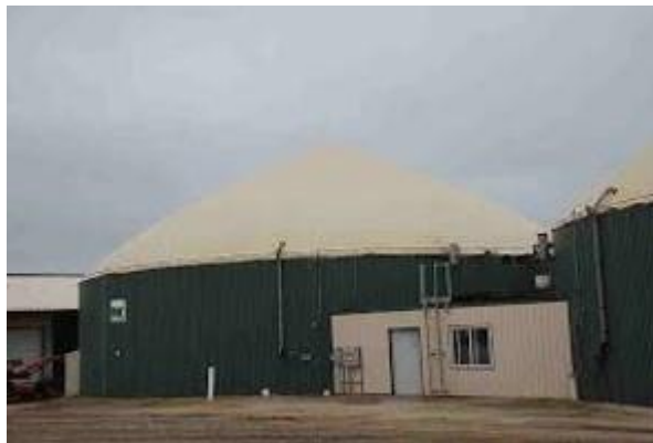
Gambar 2.4 Biodigester Complete Mix (Sumber: M Rizky, ITB 2014)
