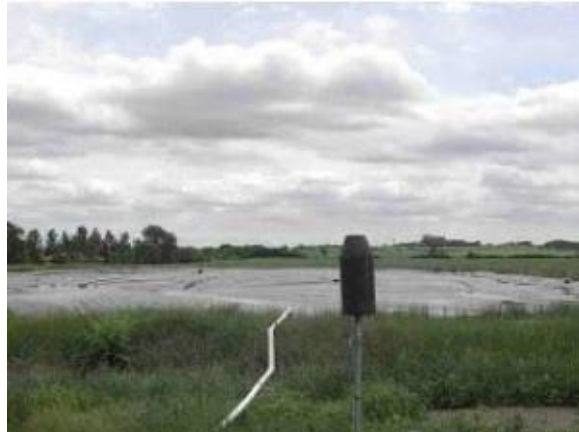
Gambar 2.5 Biodigester Cover Lagoon (Sumber: M Rizky, ITB 2014)
