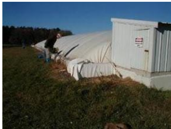
Gambar 2.6 Biodigester Plug Flow (Sumber: M Rizky, ITB 2014)
