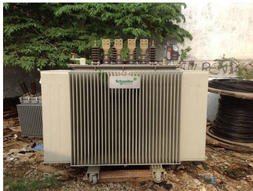
Gambar 2.5. Transformator Step-down
