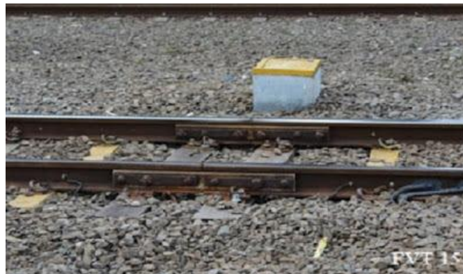
Gambar 5.2 Penampang Fish Plate
