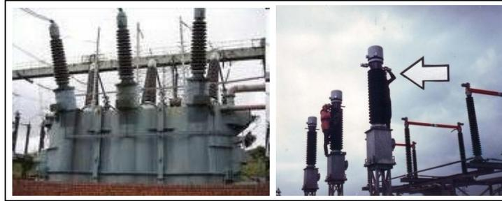
Gambar 2.4. Trafo Arus { *Current Transformer (CT)* }.
