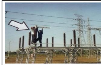
Gambar 2.5. Sakelar Pemisah (PMS) {*Disconnecting Switch (DS)*}.
